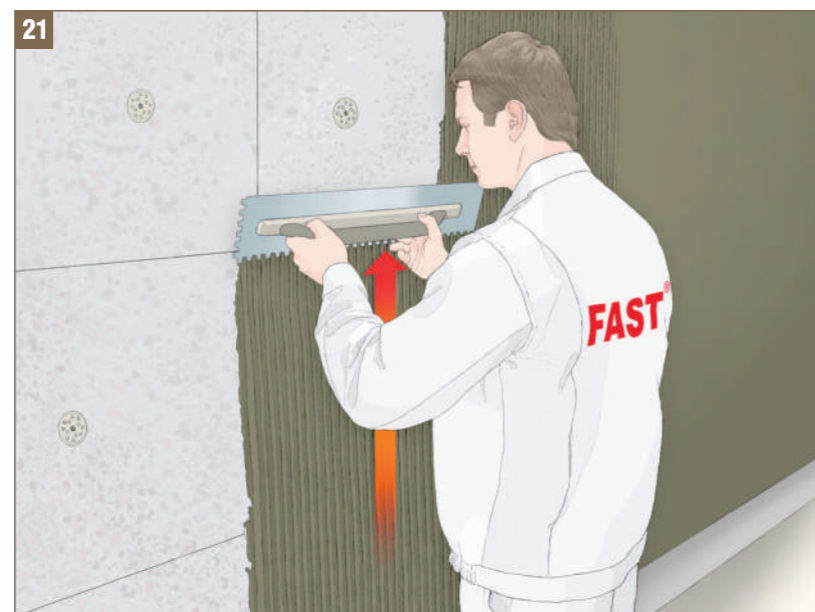
Fig. 21 - Applying mortar glue using notched trowel
