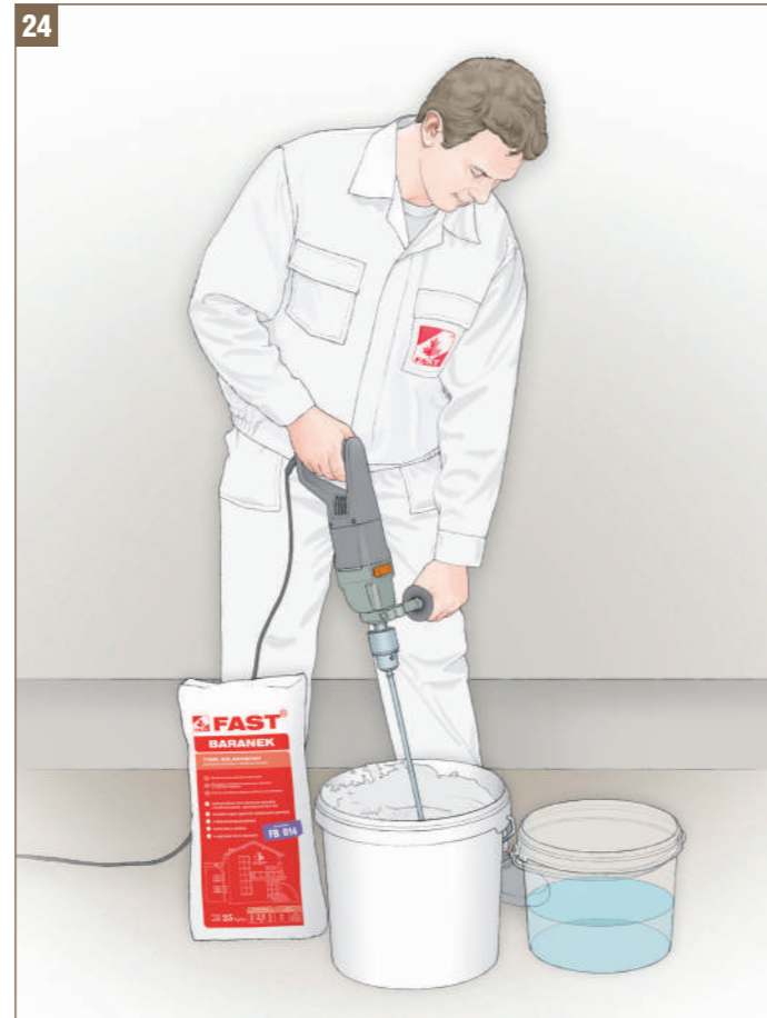
Fig. 24 - Preparation of plaster prior to application (polymer-mineral plasters)
