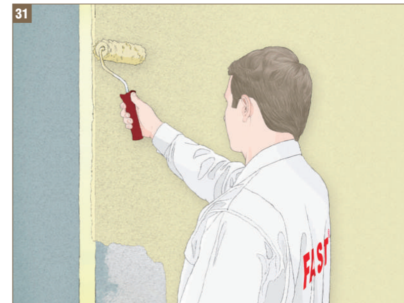
Fig. 31 - Painting plaster © FAST 2008
