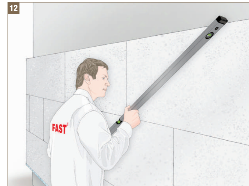
Fig. 12 - Checking board flushness after fixing © FAST 2008
