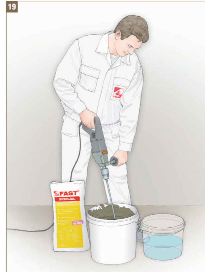
Fig. 19 - Preparation of FAST SPECJAL mortar glue © FAST 2008
