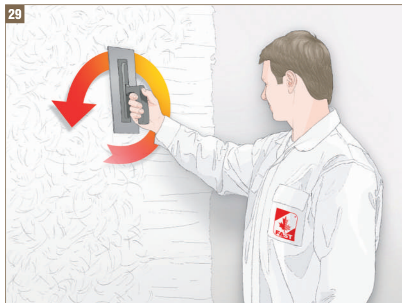
Fig. 29 - Giving texture to plaster - swirl grated structure © FAST 2008
