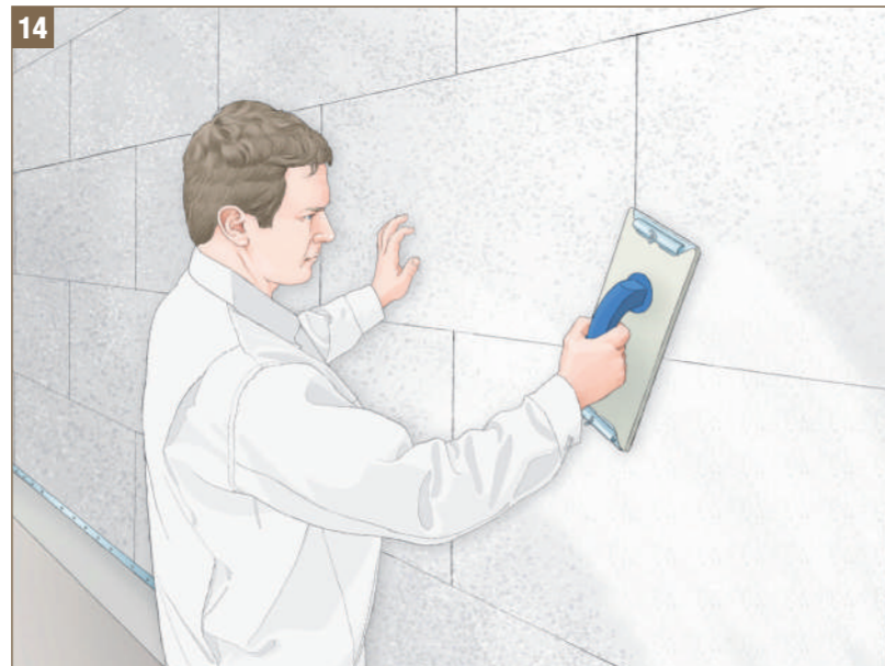
Fig. 14 - Leveling plane through grinding © FAST 2008
