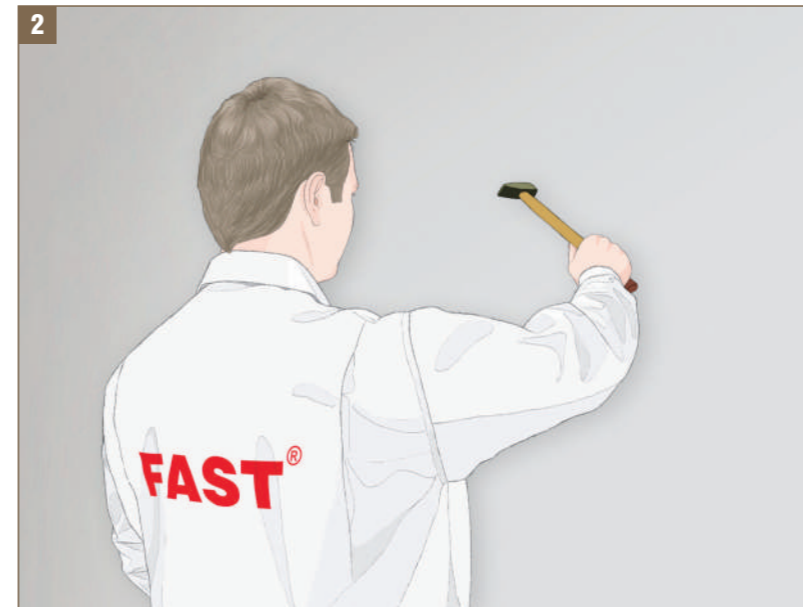
Figure 2 - Checking the surface by tapping
