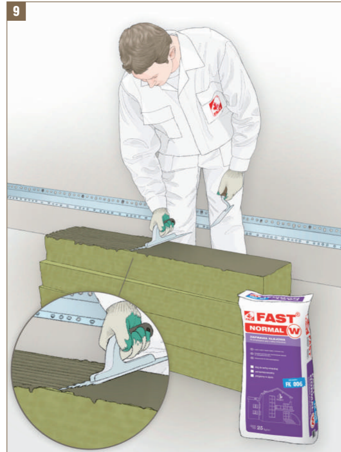
Fig. 9 - Applying mortar glue to lamella mineral wool panels © FAST 2008
