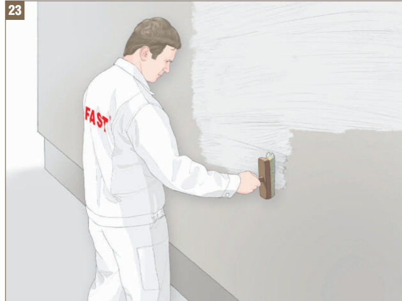
Fig. 23 - Applying the undercoat
