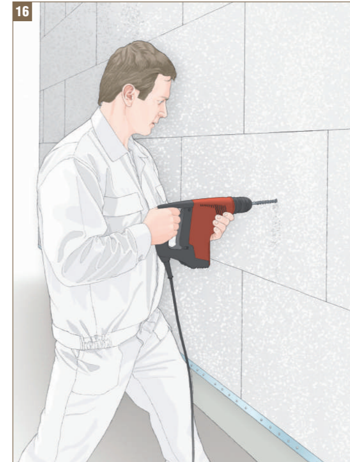
Fig. 16 - Drilling holes for mechanical fixings © FAST 2008
