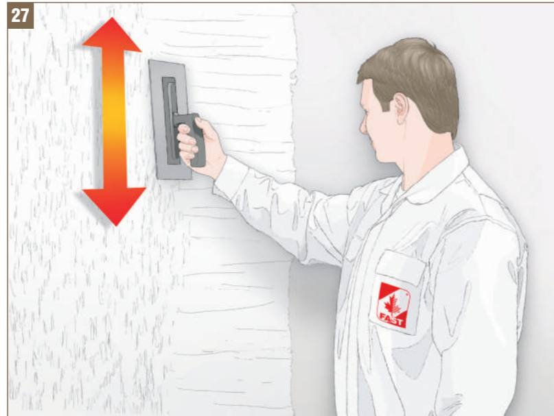
Fig. 27 - Giving texture to plaster - vertical grated structure © FAST 2008
